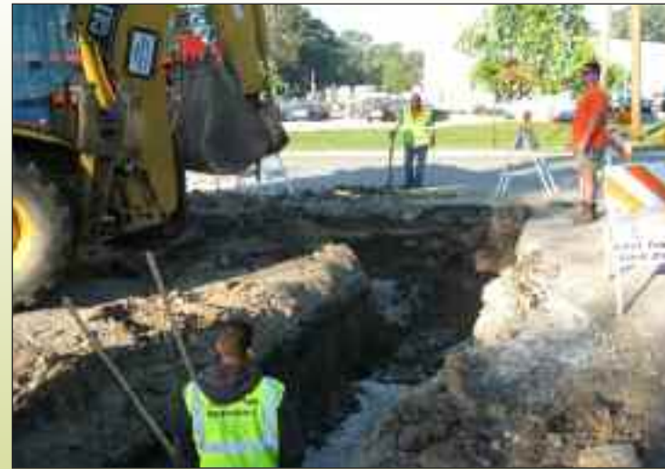
Township Road District Employees working on drainage ditch improvements.
