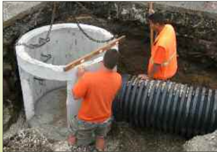
Foreman Eric Baranak and laborer Jaime Guajardo installing a storm sewer catch basin.
